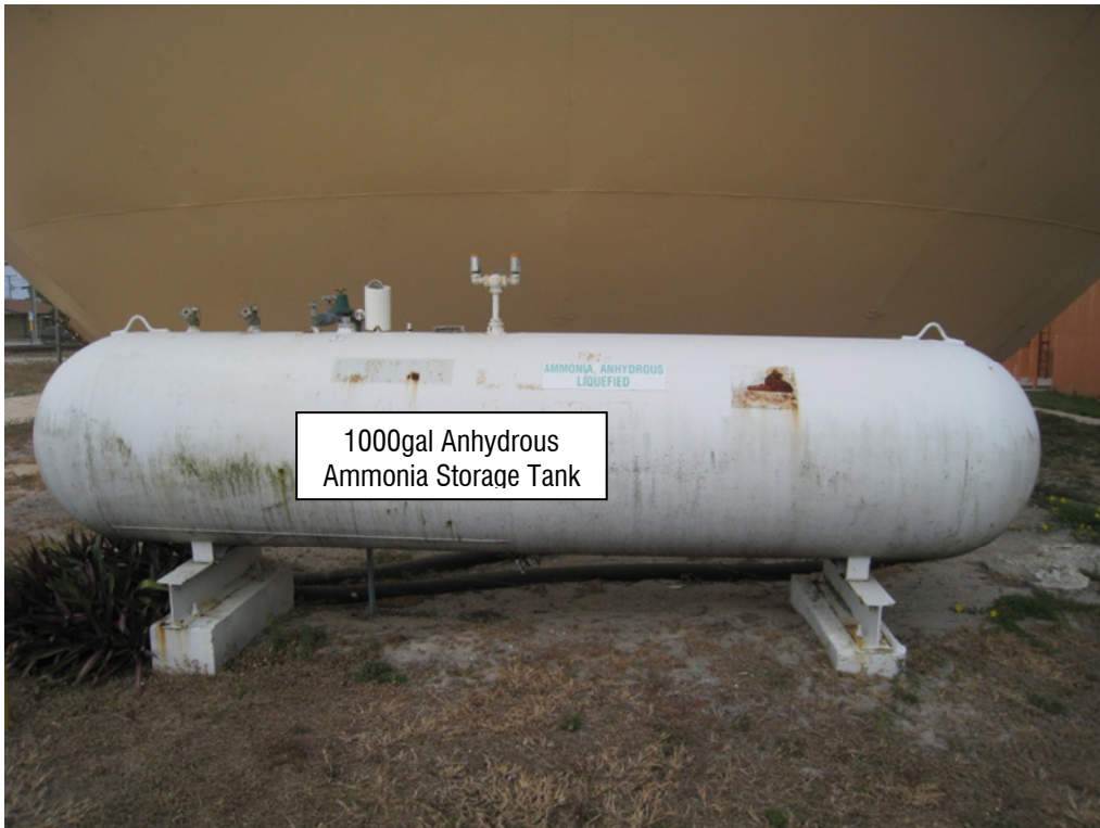
Picture A.8-1 1000 gallon Liquefied Anhydrous Ammonia Storage Tank
