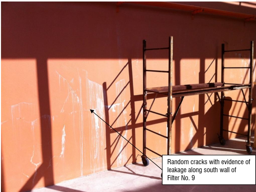
Picture A.11.9 Exterior South wall of Filter No. 9
