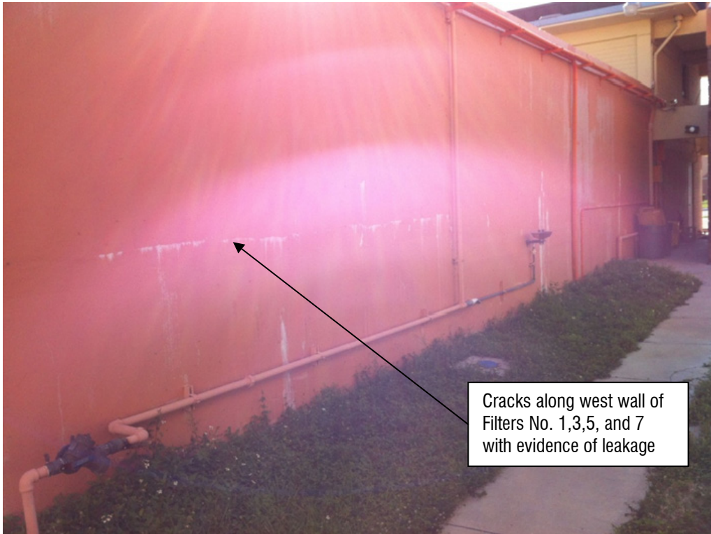
Picture A.11.4 Exterior West wall of Filters No. 1,3,5, and 7
