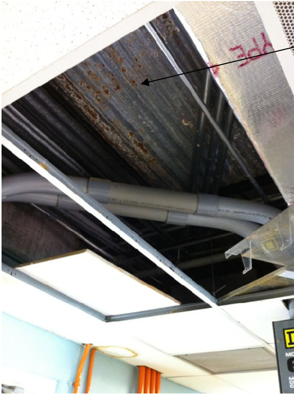
Picture A.16.1 Roof Leak above Main MCC Room
