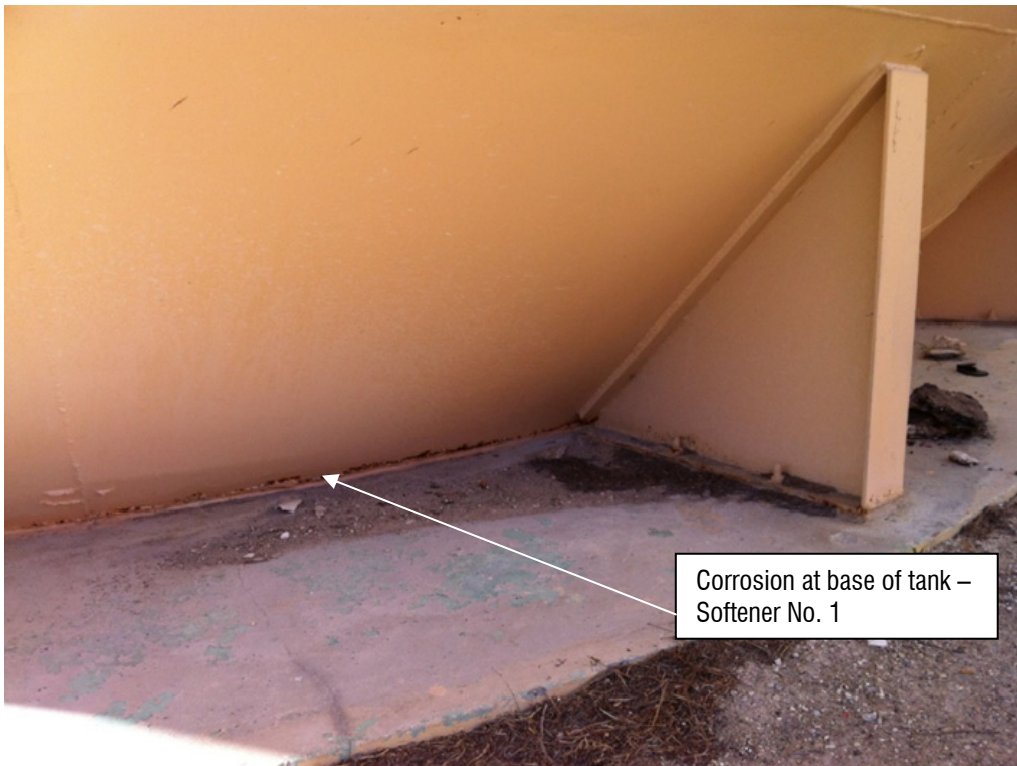
Picture A.9-6 Softener No. 1 Base of Tank
