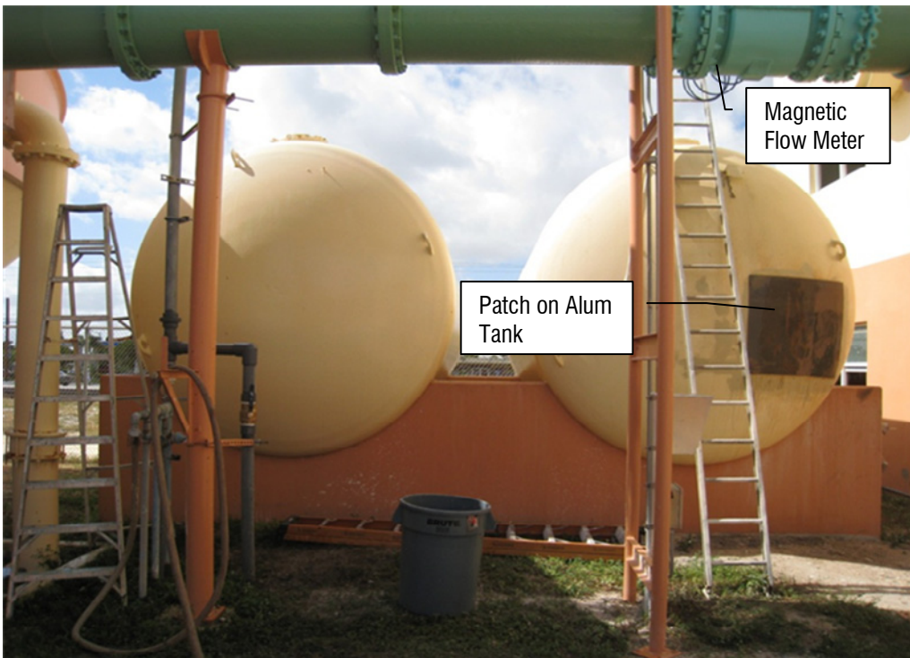
Picture A.5-1 Alum Storage Tanks and Magnetic Flow Meter (Softener No. 1)
