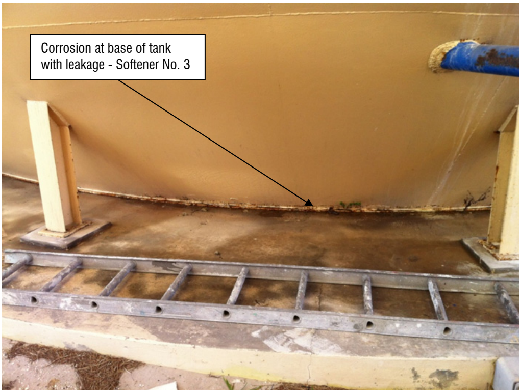
Picture A.9.7 Softener No. 3 Base of Tank
