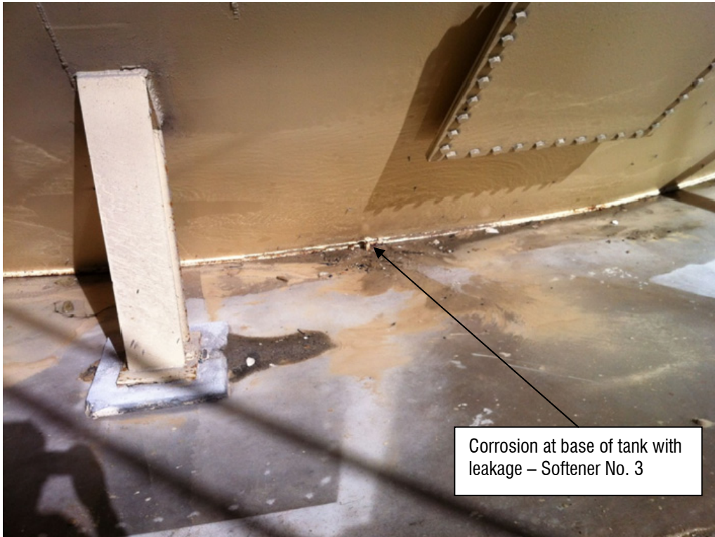
Picture A.9.8 Softener No. 3 Base of Tank
