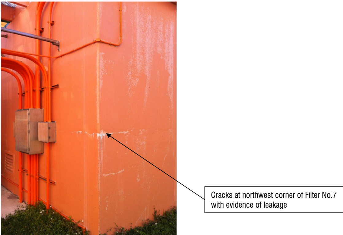
Picture A.11.5 Exterior Northwest wall of Filter No. 7
