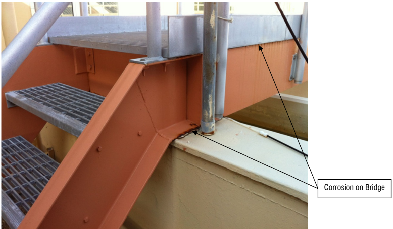
Picture A.11.3 Bridge Corrosion on South Filter Bank
