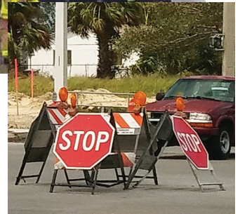
Portable stop signs used to make four-way stops due to power outages
