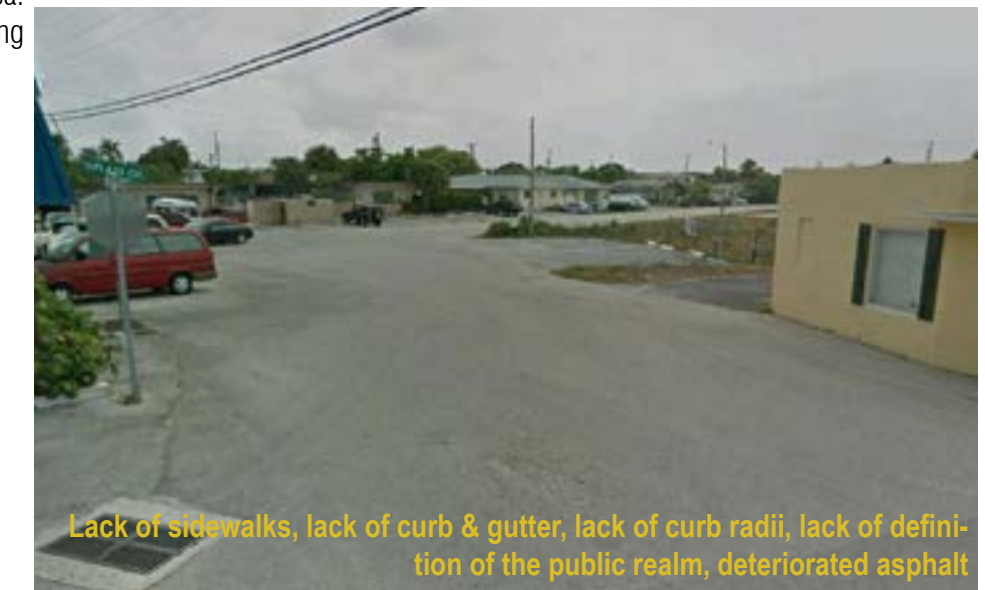
Lack of sidewalks, lack of curb & gutter, lack of curb radii, lack of definition of the public realm, deteriorated asphalt
