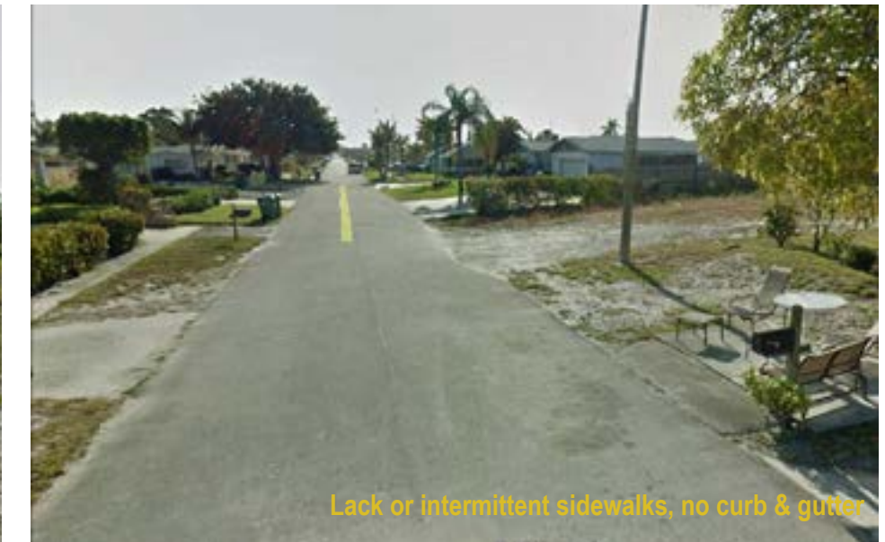
Lack of sidewalks, curb & gutter
